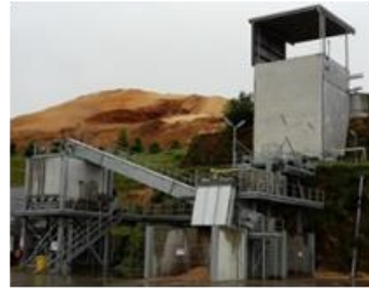
Product screened for metal & oversize before drying
